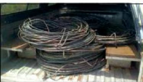
Stolen copper cables recovered by the cable theft task team
